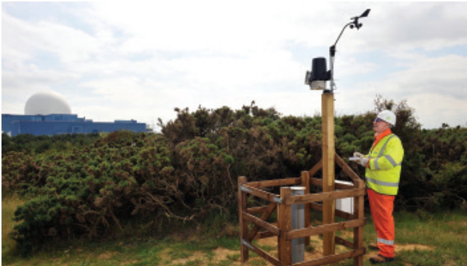
Investigative work currently taking place on the Sizewell C development site
